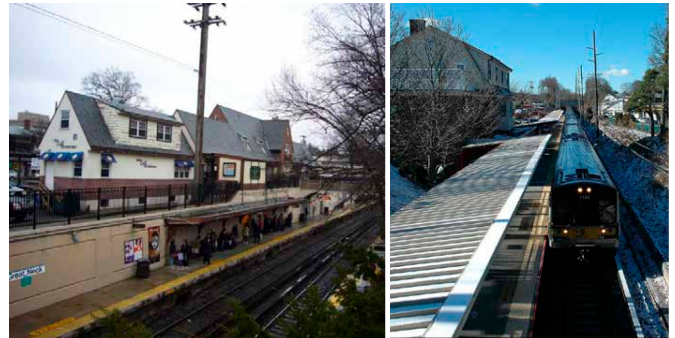
Great Neck, left, and Manhasset, right, have tracks depressed below grade level.
