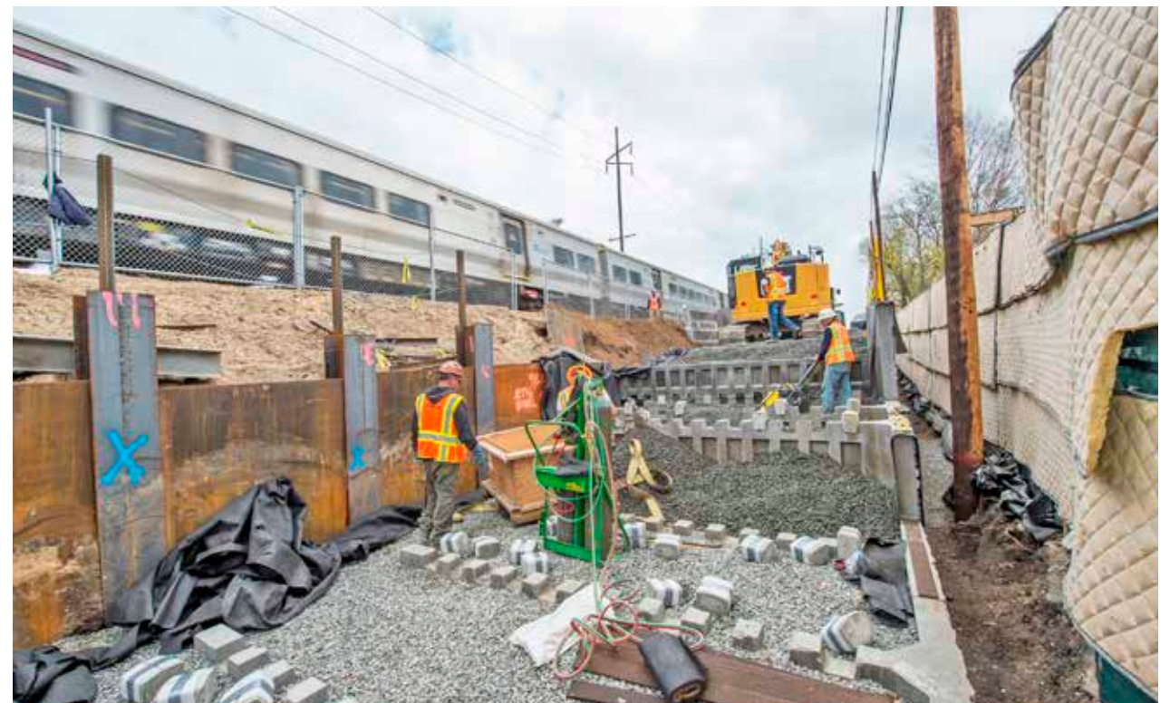
Sound and retaining walls under construction. Nearly nine miles of such walls will be built in the project area. © Metropolitan Transportation Authority
